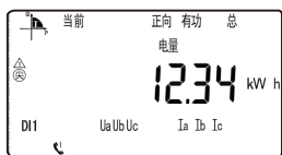
Current forward active energy 12.34kWh
